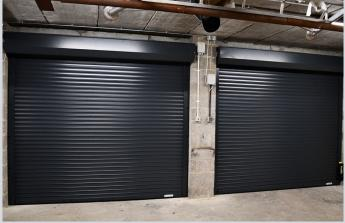
The product was a Xonar 943 with an upgraded anti-cut core to stop powered cutting equipment penetrating the shutter. The Xonar only needs a small space for rolling the shutter curtain and it was fitted with unique self-locking technology.
